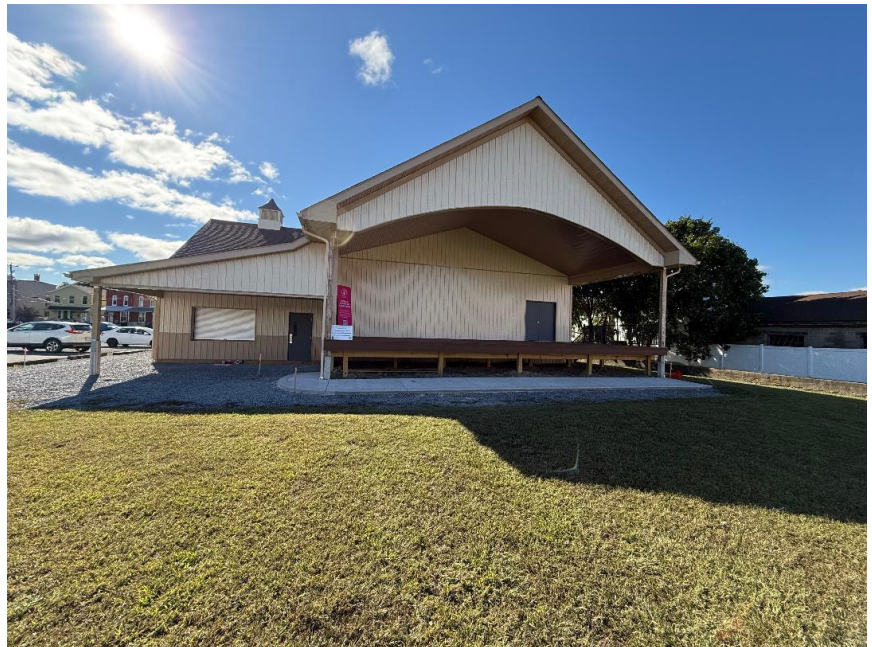
Completed façade and stage at State Street Square.
